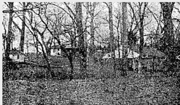
Paroquet Springs fishing camp with cabins, ice house, kitchen/dining hall
